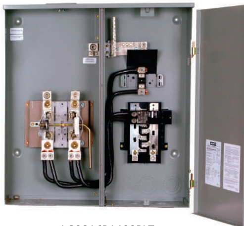
LG0816B1400RLT 8 space, 10 circuit feed thru lugs
