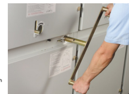
Figure 7-5 Earthing switch operation
