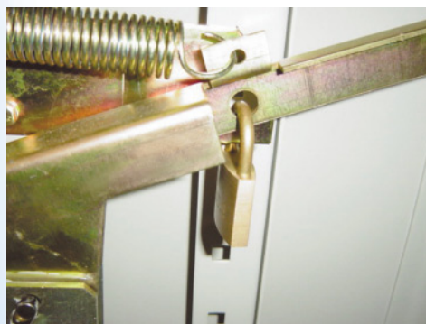
Figure 4-8 Optional padlocking of top and bottom shutters
