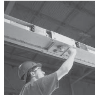
Typical Busway Installation (Torque Indicating Bolt)
