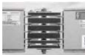
Bridge Joint Assembly
