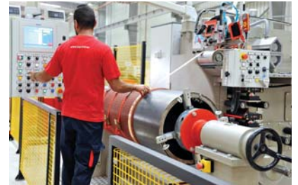
HV strip winding machine.
